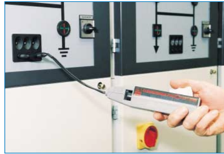
Testing the LED voltage indication.
