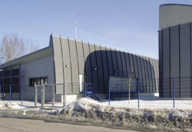
Innovac MMS power distribution, Kivenlahden, Espoo, Finland
