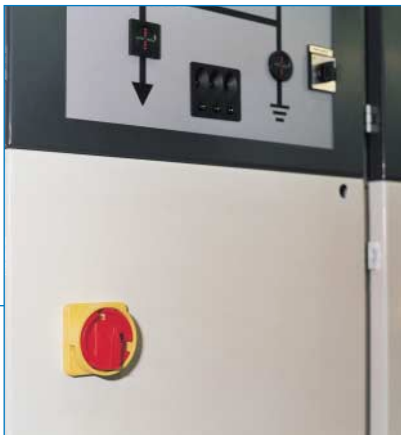
Operating switch with padlocking feature (optional).
