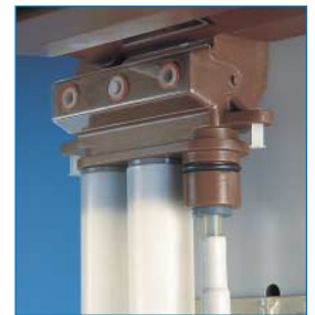
Transformer connection for Magnefix type MF.
