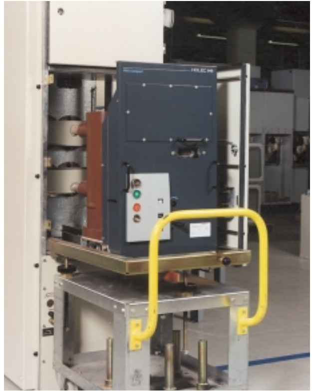
HOLEC vcb in 620 mm wide panel of Holec Unitole MV switchboard
