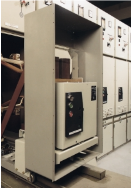
Refurbishment for Main Oil Terminal, Rotterdam of 2 MV switchboards
