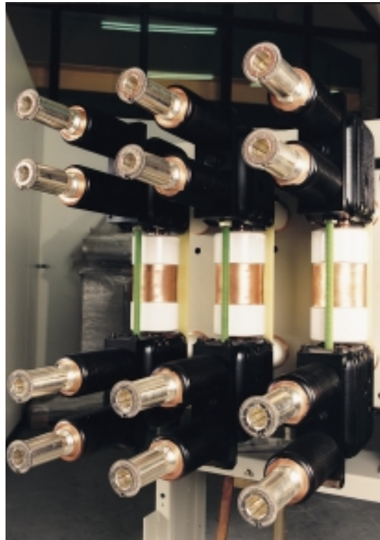
Holec is your partner in electrical power engineering
